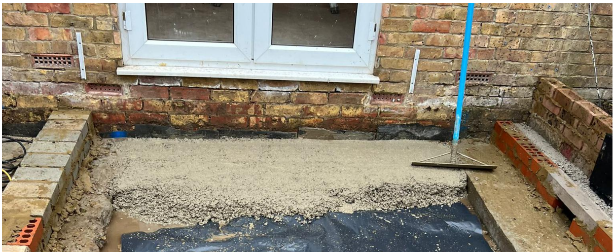
Dug down and added membrane then 4 inches of concrete (similar to old conservatory)
