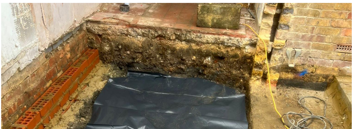
Dug down and added membrane then 4 inches of concrete (similar to old conservatory)
