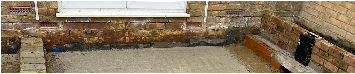
Concrete added to section next to dining area
