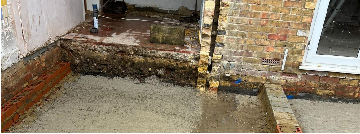
Concrete added to section over original kitchen next to utility area
