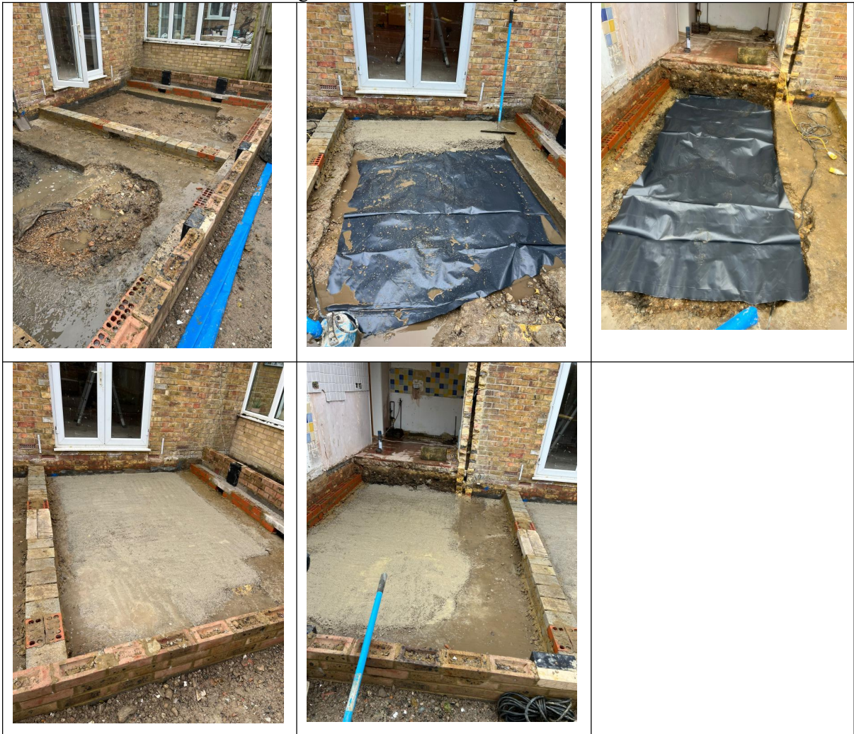
Concrete added to section over original kitchen next to utility area
